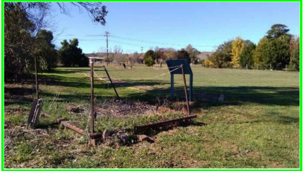
Photo #5 – Remains of Well Block
