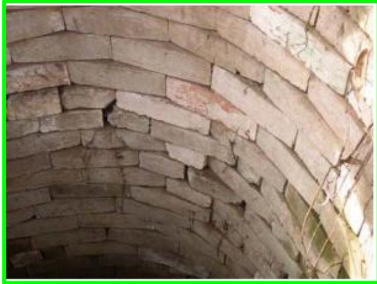
Photo #6 – Interior of Well
